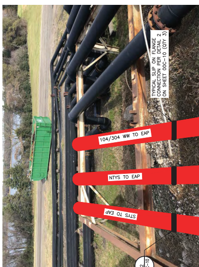
TERMINATION DETAIL C AT EXISTING PIPE RACK (C) 00C-09 NOT TO SCALE
